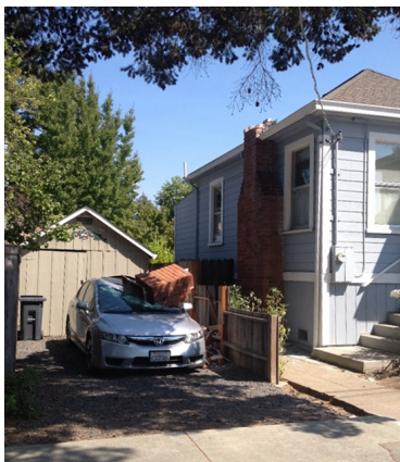
Louay Shamroukh | South Napa Earthquake Clearinghouse, EERI
